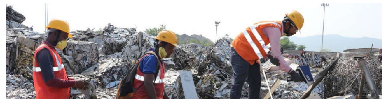
Material Management: Sorting through high value material from lean scrap
